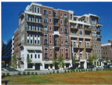
The Bookends, an eight-story mixed use project in Greenville, S.C., includes 30 residential units and fronts a new city parking garage; the first floor has retail and commercial space.
