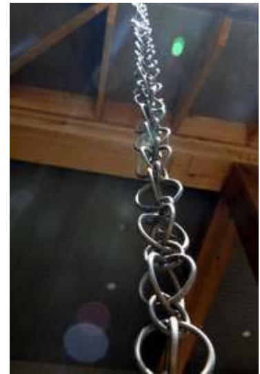
The Cliffs Cottage on the Furman University campus uses rain chains to bring roof water down that can be filtered and emptied into the lake. (HEIDI HEILBRUNN/Staff)
